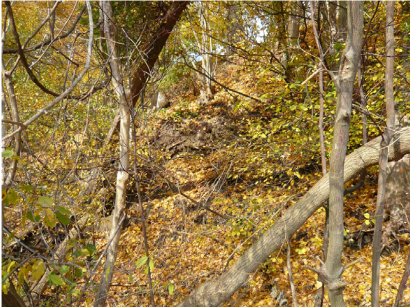
Photo 7: Slope above the crib. Portion of the slope are steep and are eroding.
