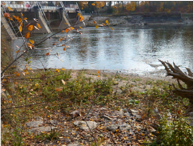
Photo 2: Downstream end of the crib, looking towards the south. Water on the bottom shows the surface runoff bypassing the downstream portions of the crib.
