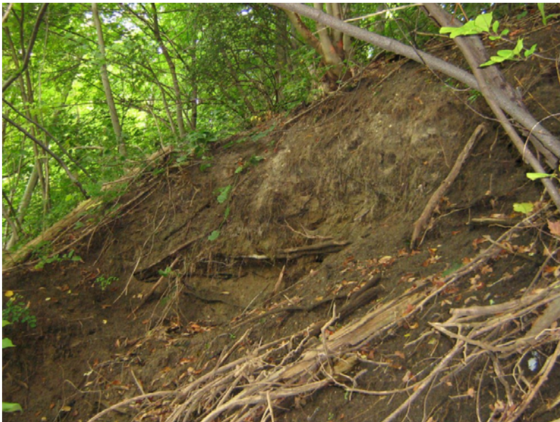
Photo 8: Slope above the crib. Slope is held together by roots, sometimes by trees that are dead.
