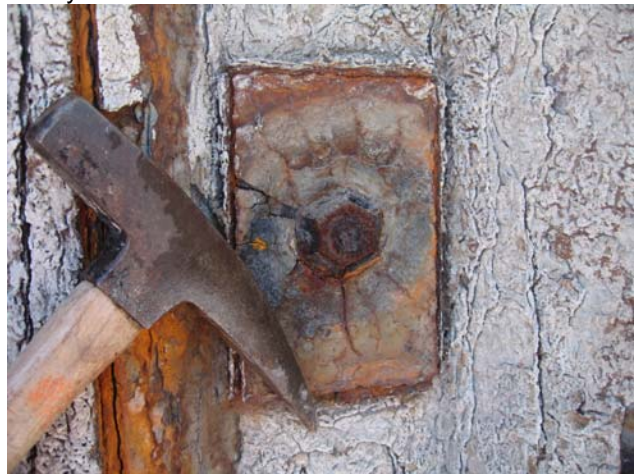
Photo #16 – Partially cleaned wale bolt assembly.
