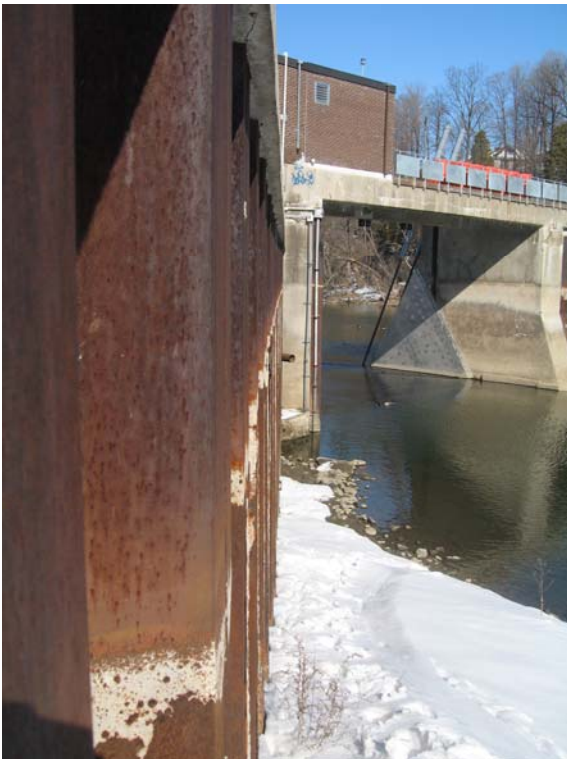
Photo #21 – Vertical alignment of face of wall, viewing west to dam
