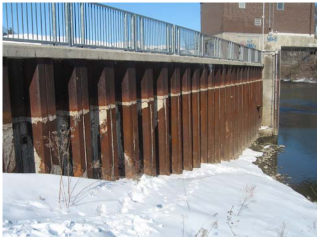
Photo #3 – Face of wall viewing west toward upstream face of dam.
