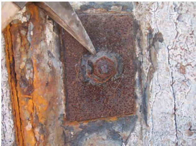
Photo #17 - Wale bolt assembly cleaned of rust scale.
