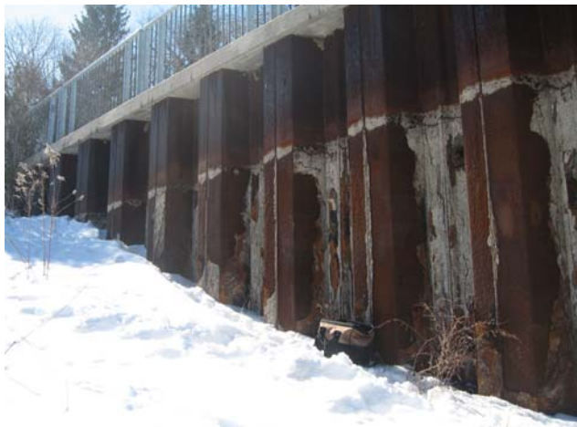
Photo #5 – Face of wall viewing east up the bank line.
