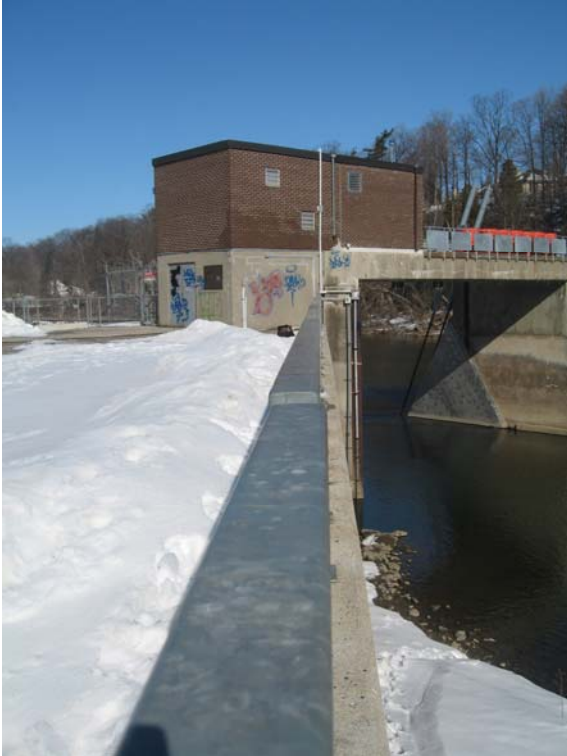
Photo #19 – Horizontal alignment of top of wall at rail height.
