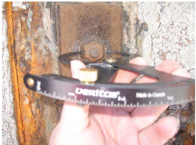
Photo #18 – Measurement across the flat of the wale bolt.
