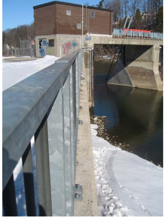
Photo #20 – Horizontal alignment of top of wall at concrete cap height.
