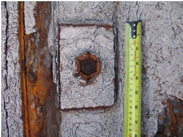
Photo #15 – Wale bolt assembly.
