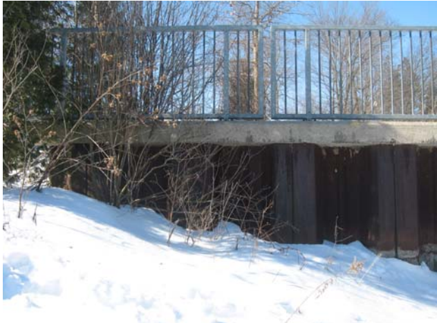
Photo #1 – Front Elevation, east end of wall.
