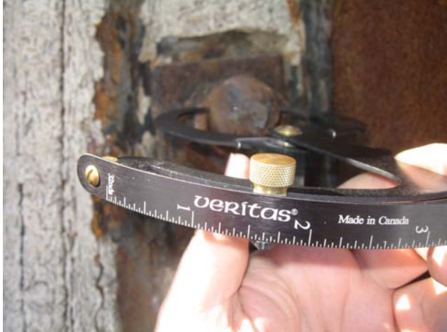
Photo #13 - Measurement across the tie rod on tie rod #7.
