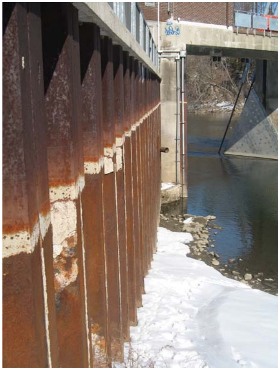
Photo #22 – Vertical alignment of face of wall along face of wall viewing west to dam.
