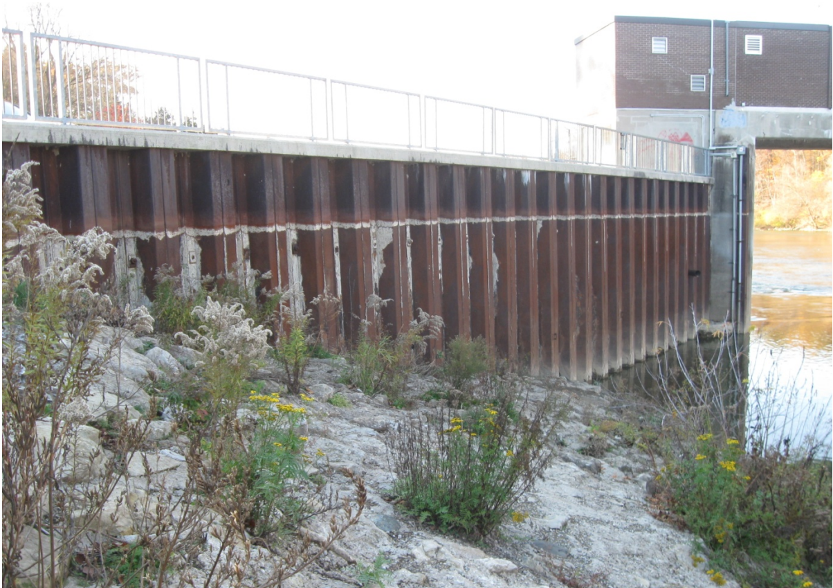
Photo 14 – Southeast steel sheet piling retaining wall
