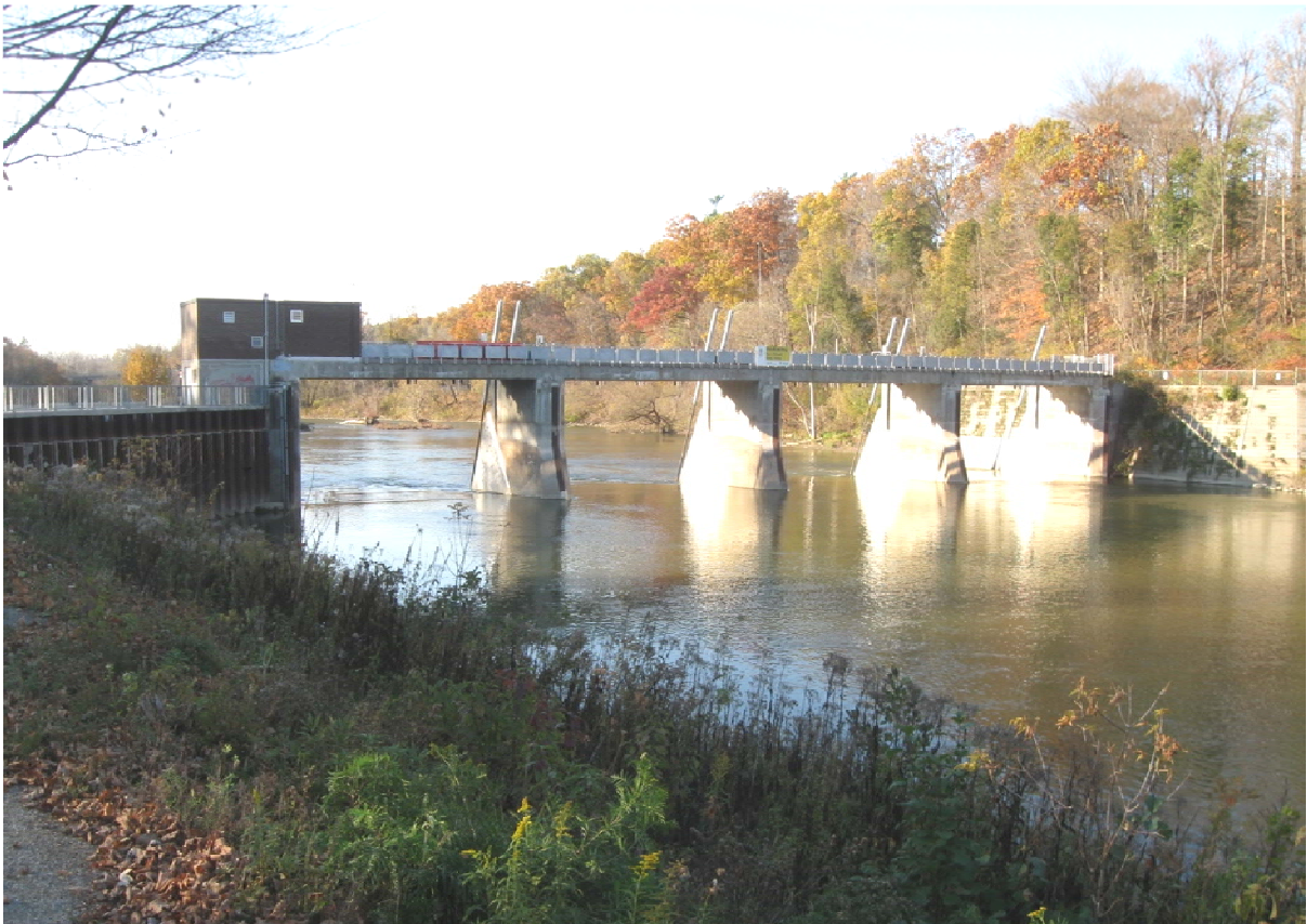
Photo 1 – Upstream of dam
