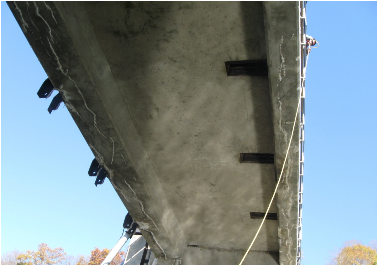
Photo 10 – Soffit of 2 nd span from south end
