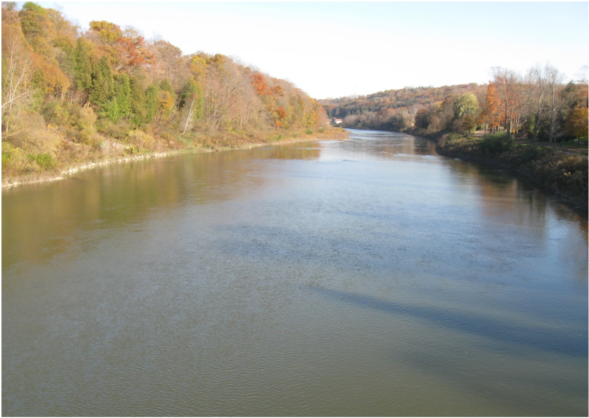
Photo 3 – Looking upstream of the dam
