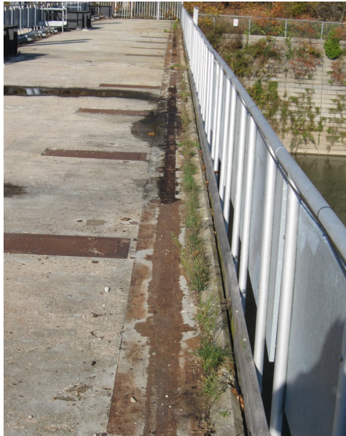
Photo 23 – East side of deck, looking north
