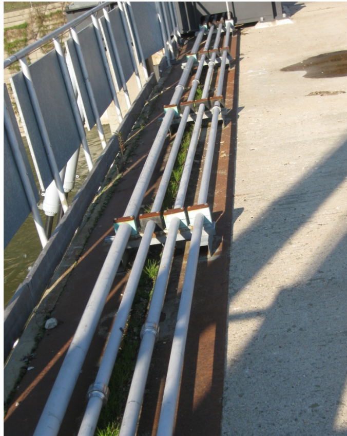
Photo 24 – West side of deck, looking north
