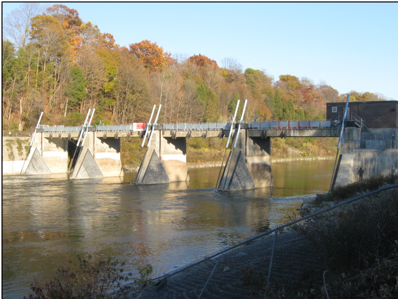
Figure 1 – General Overview of the Springbank Dam
