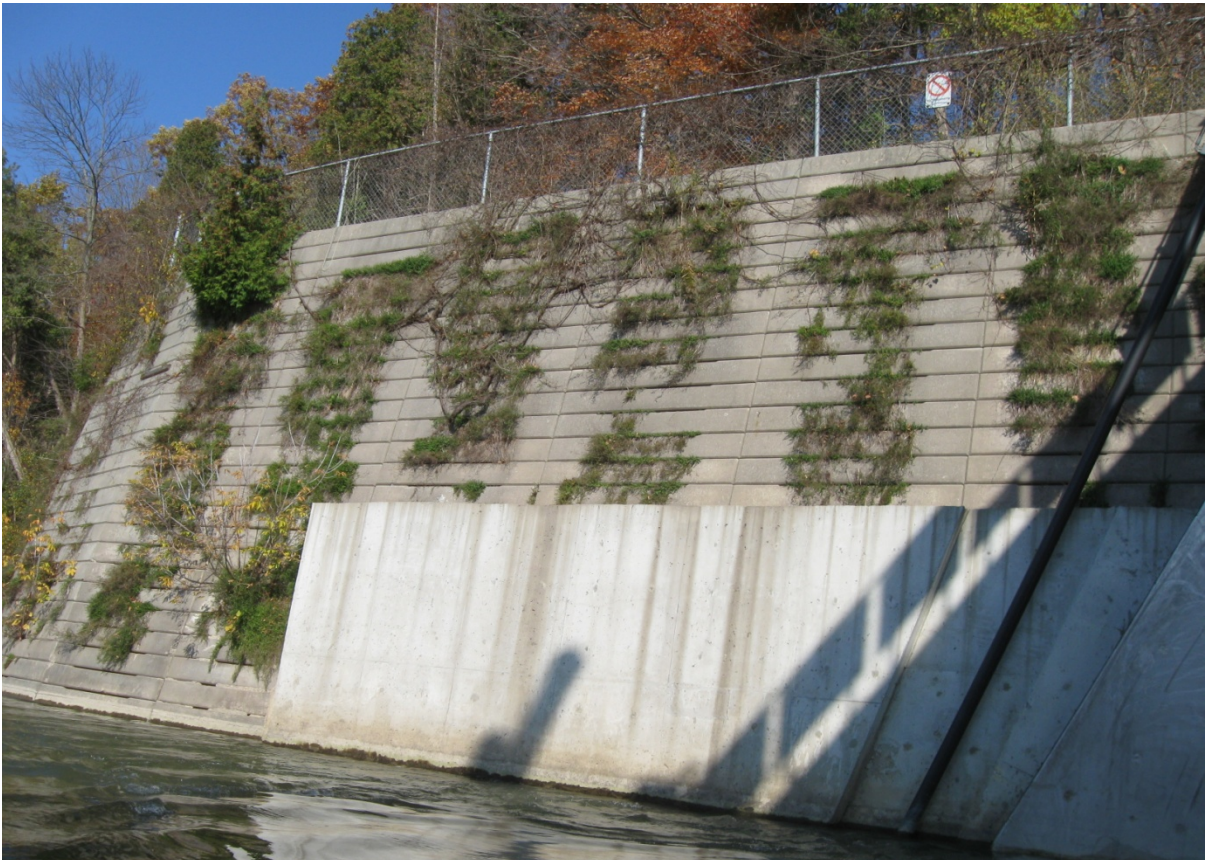
Photo 15 – Northwest retaining wall
