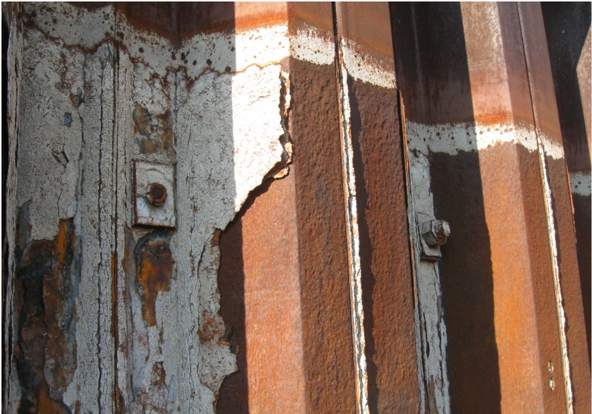
Photo 28 – Vertical surface of southeast retaining wall
