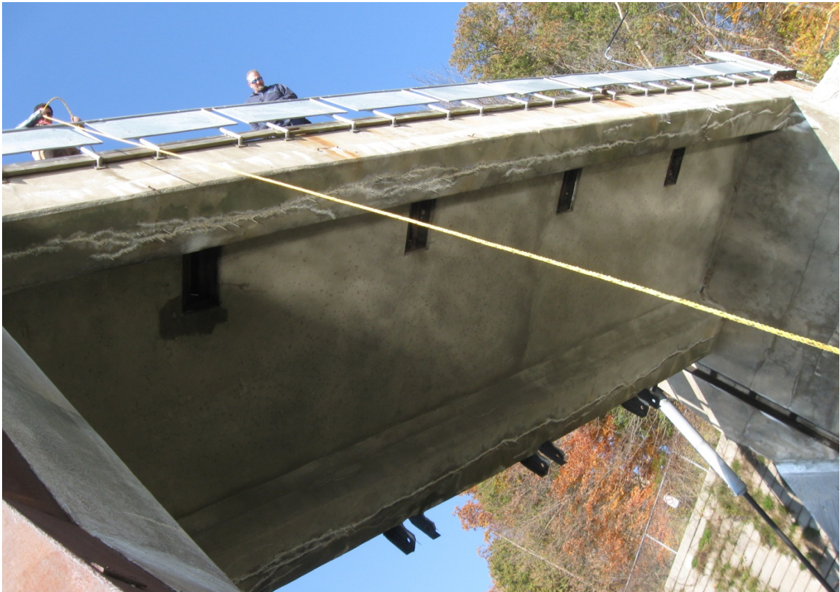
Photo 12 – Soffit of north span
