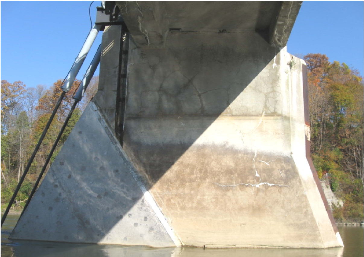
Photo 21 – Typical pier condition, south elevation of south pier
