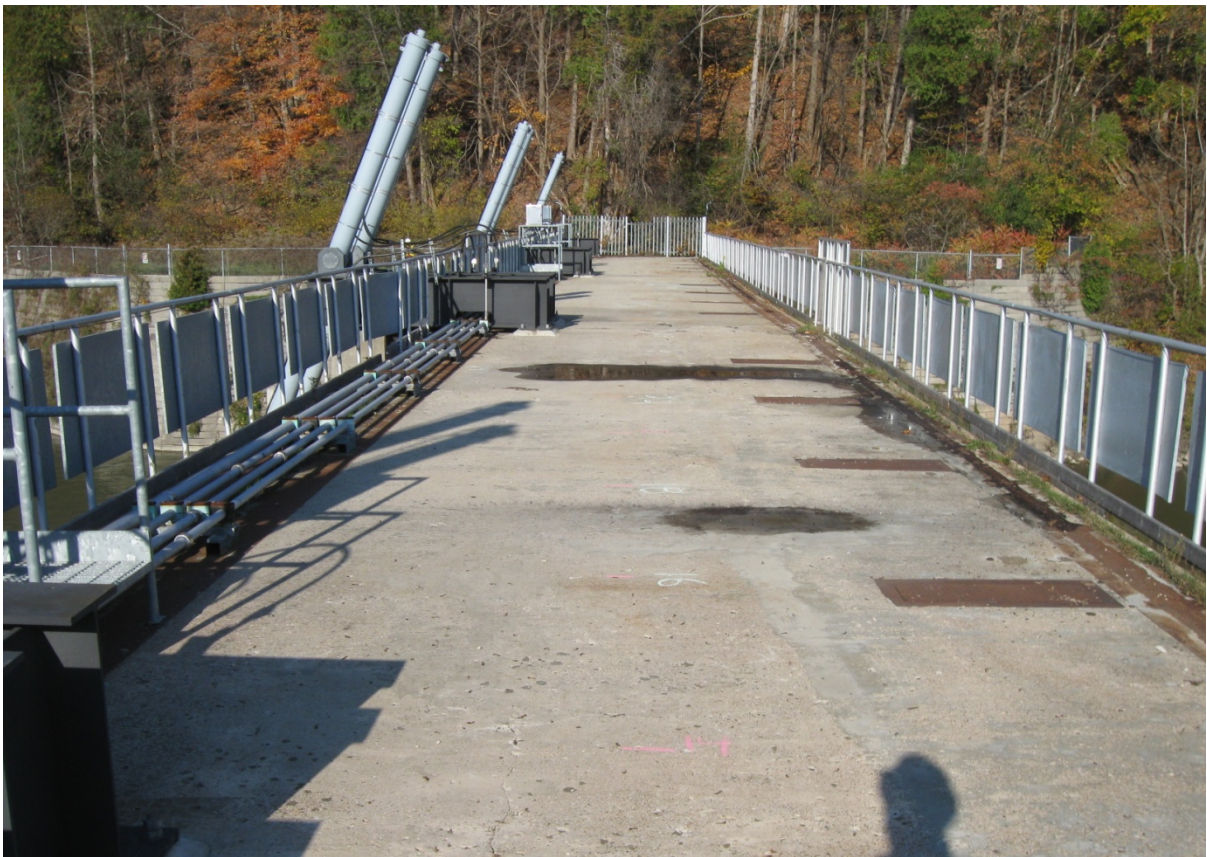
Photo 5 – Deck, looking north
