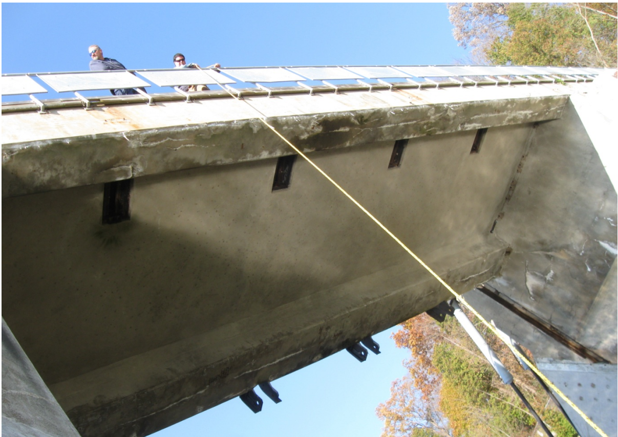
Photo 11 – Soffit of 2 nd span from north end
