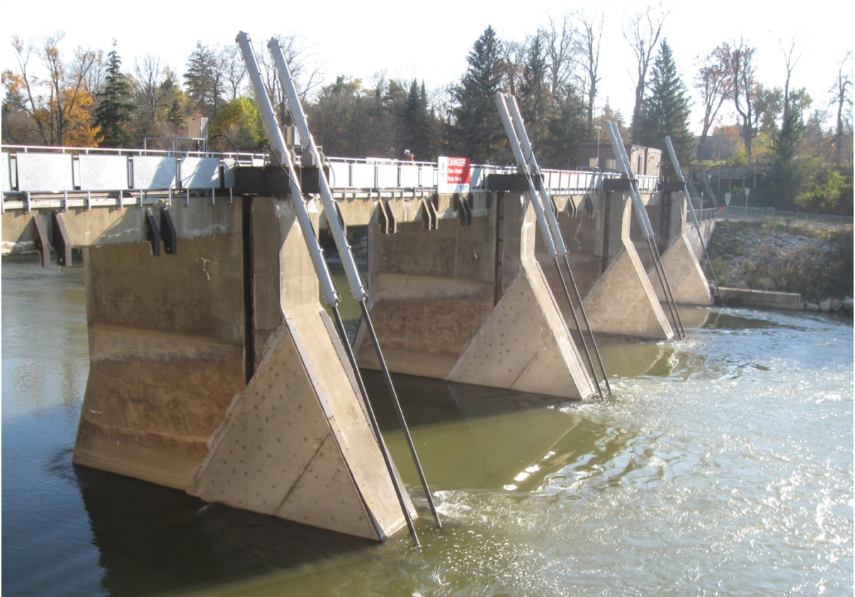
Photo 20 - Downstream piers, looking south
