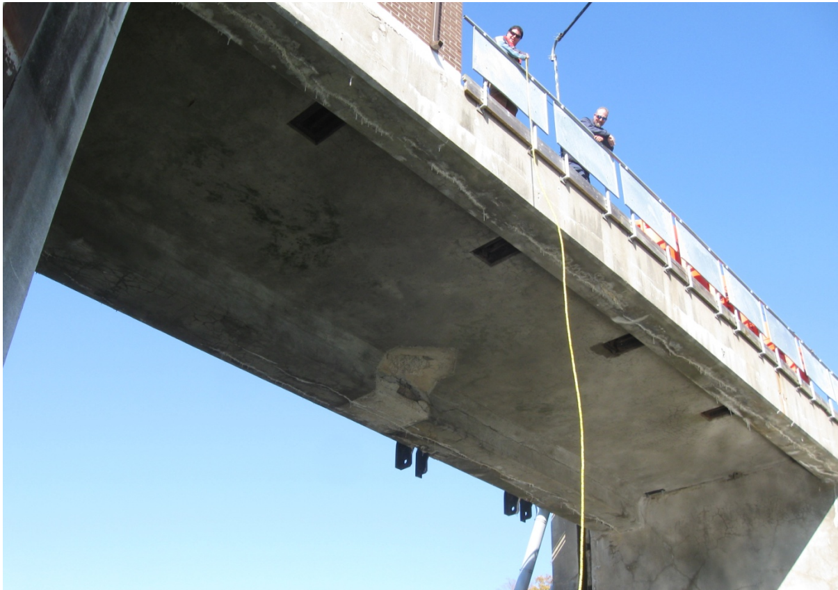
Photo 8 – Soffit of south span
