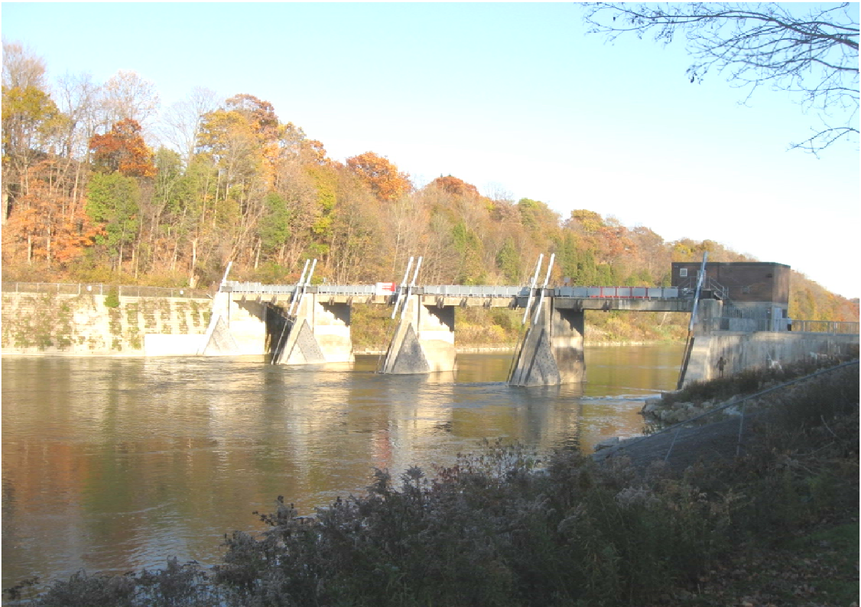
Photo 2 – Downstream of dam
