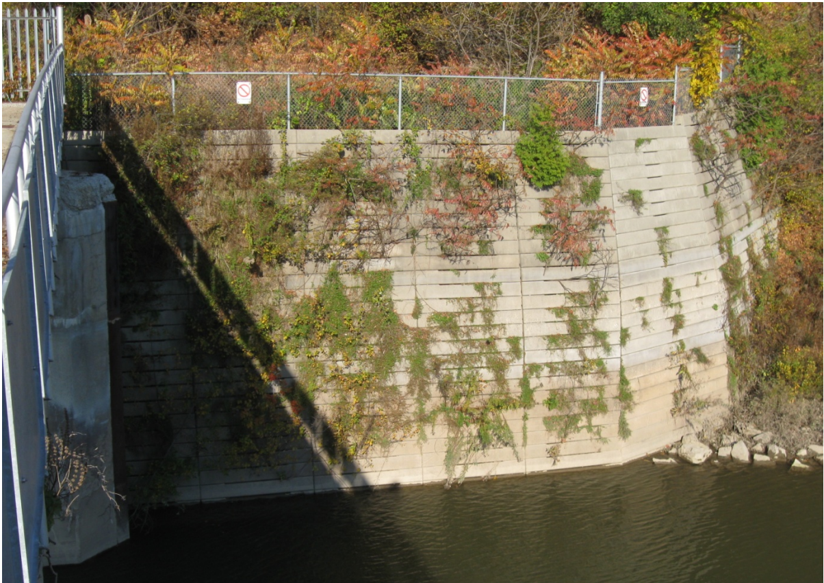
Photo 13 – Northeast retaining wall
