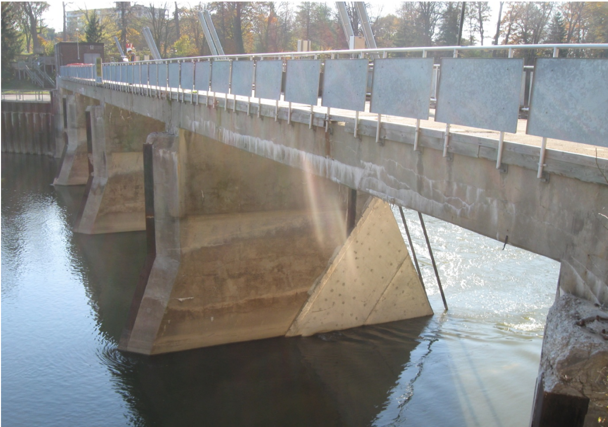
Photo 18 – Upstream piers, looking south
