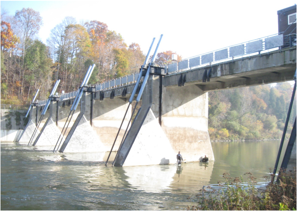
Photo 19 – Downstream piers, looking north
