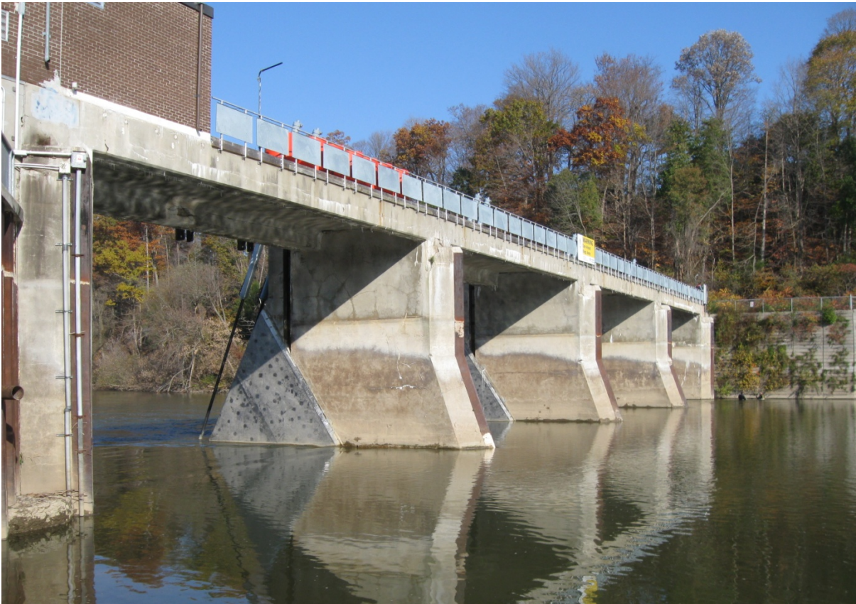
Photo 17 – Upstream piers, looking north
