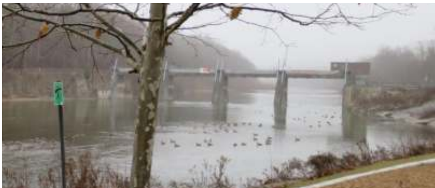
The rebuilt Springbank Dam, fall 2014. UTRCA photo.
