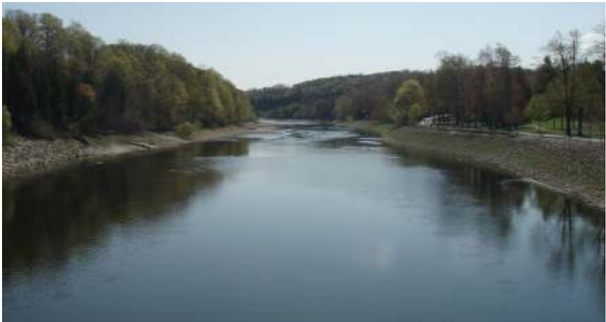
Photo 4. April 30 th , 2008 looking upstream from Springbank Dam. Photo by John Schwindt
