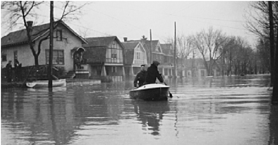
Floods on Wharncliffe Road (1937).
