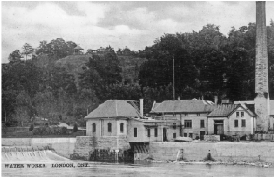
Waterworks at Springbank
