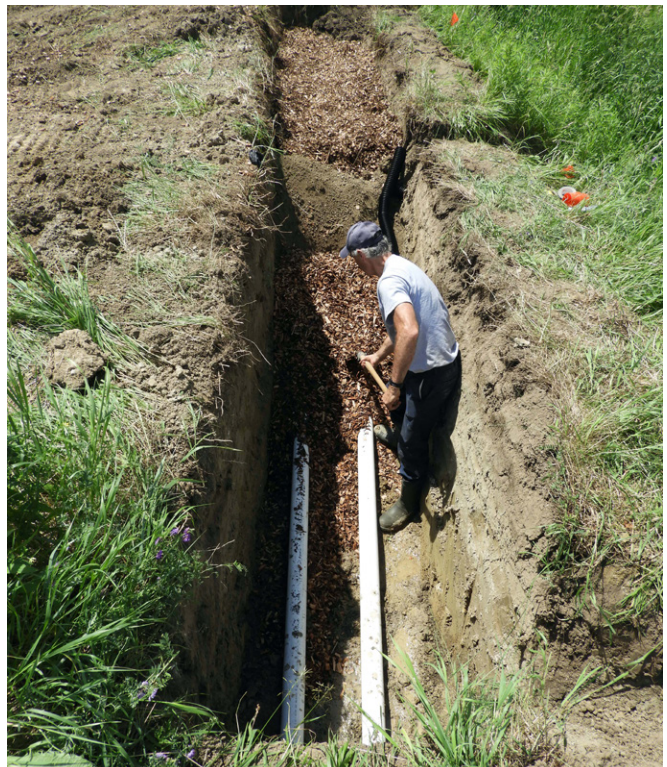
Staff install a woodchip biofilter.
