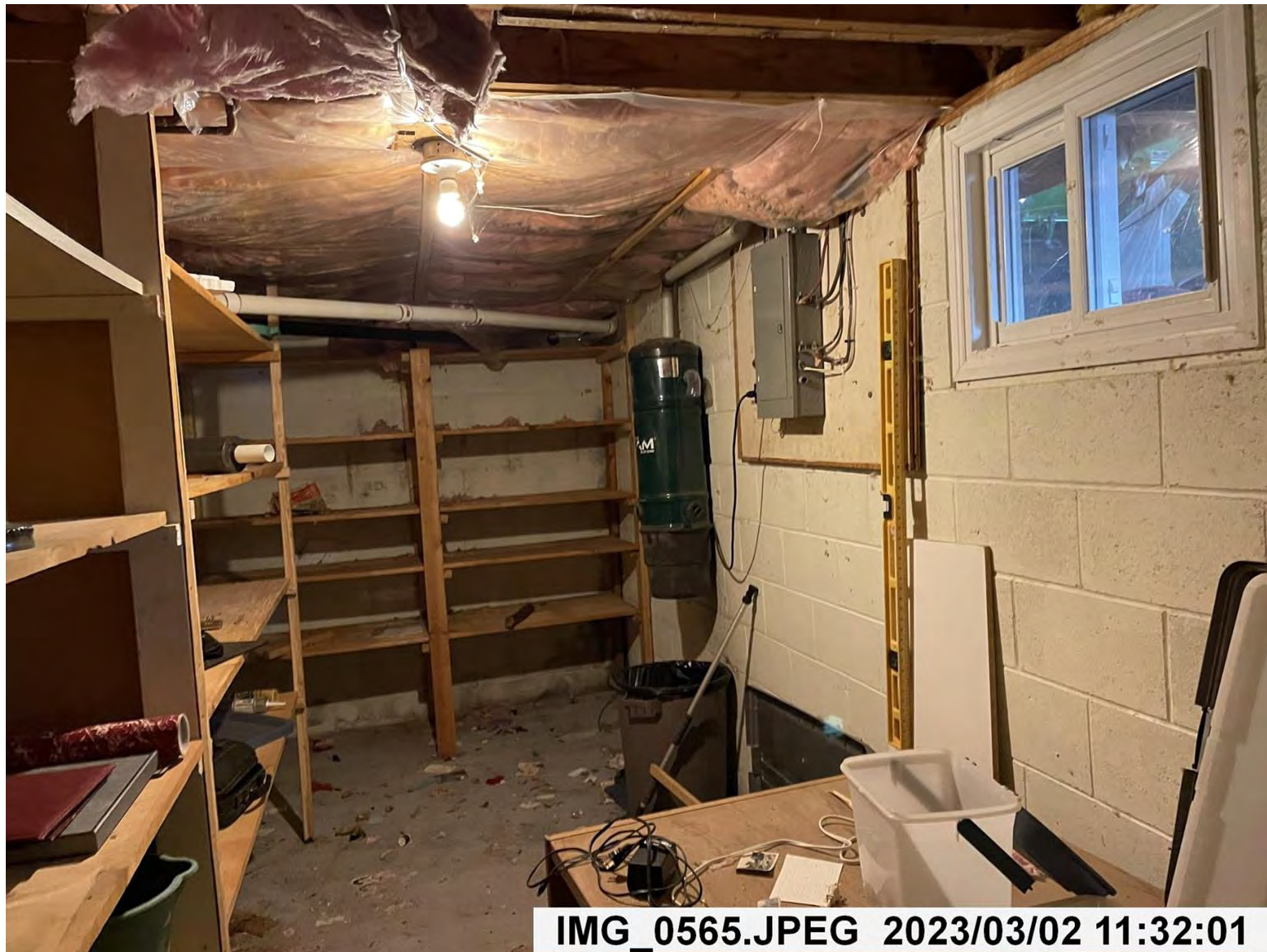
Utility/storage room in basement
