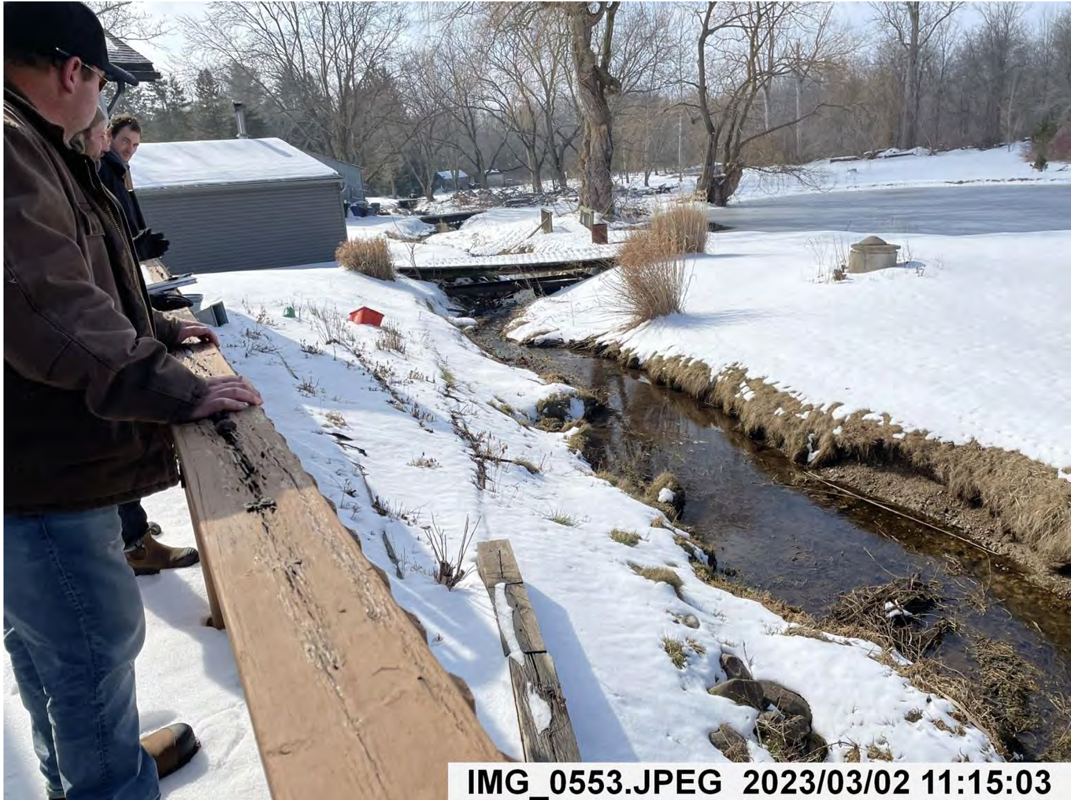
Looking downstream (S) of Benfield Drain from deck at W of house
