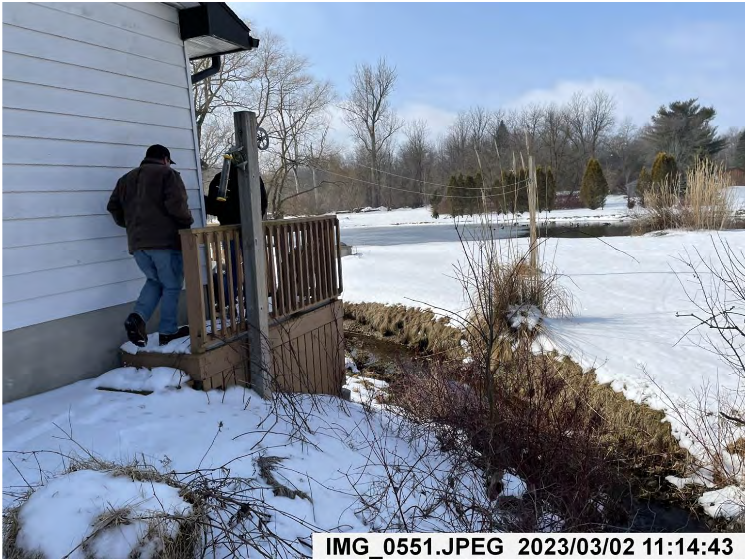
Deck access at NW corner of house, Benfield Drain downstream
