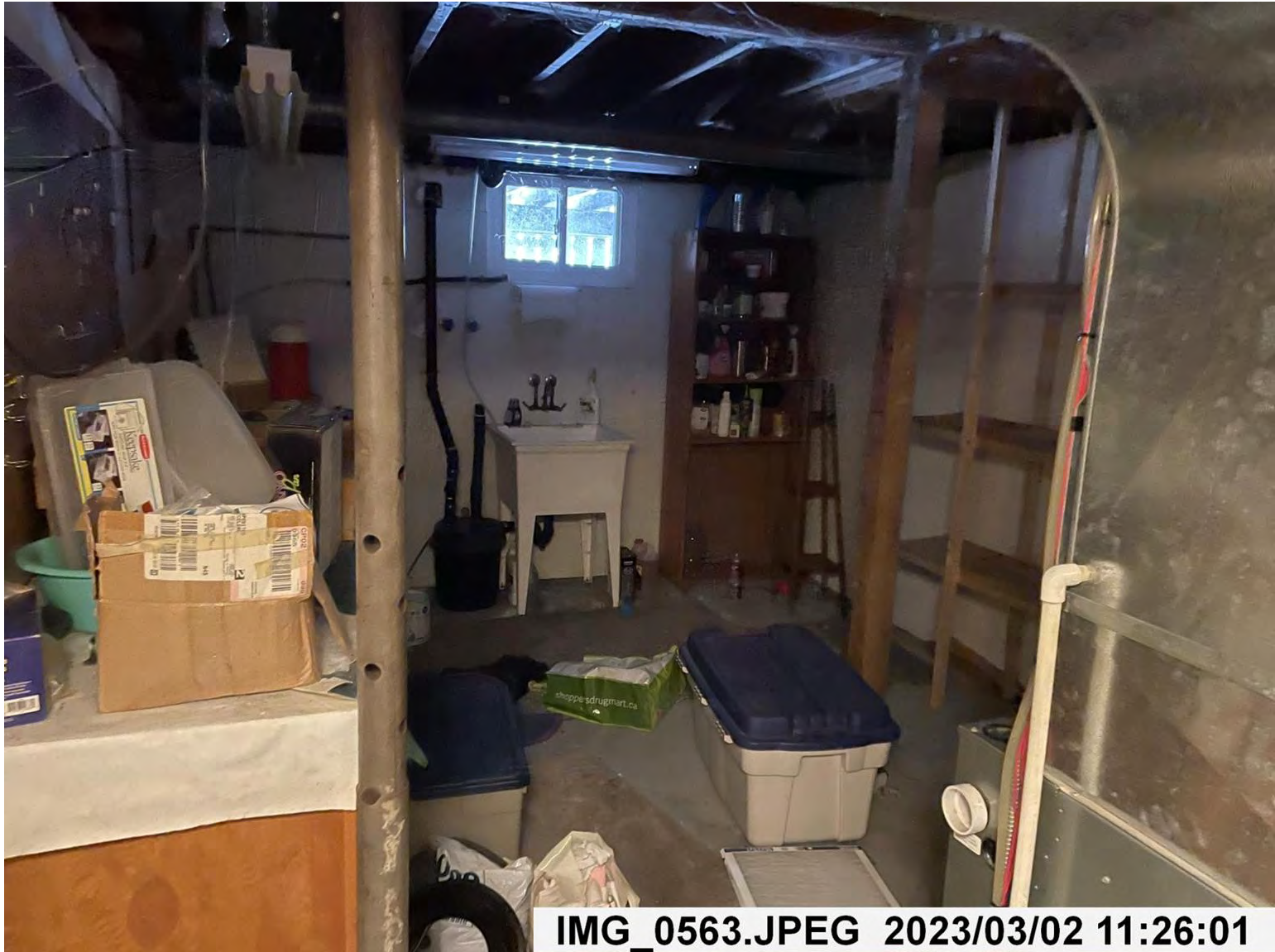
Utility/storage room in basement
