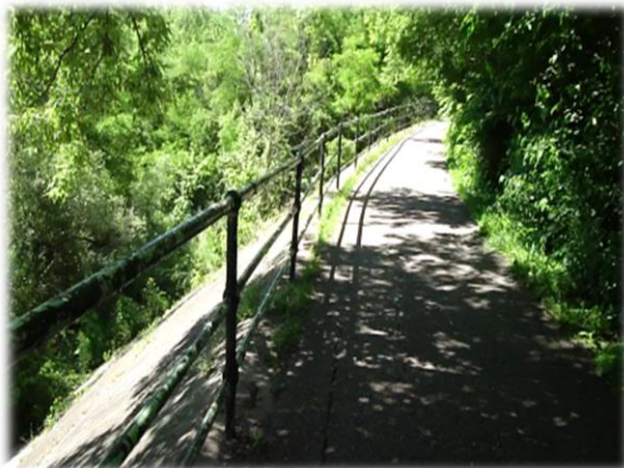
Figure 4.10: Natural Bank (South of Bridge, Facing South)
