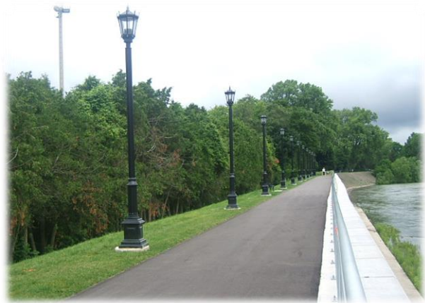
Figure 7.6: Phase 1 Light Post
