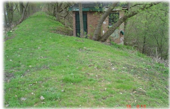
Figure 4.23: Douglas Avenue Pumping Station
