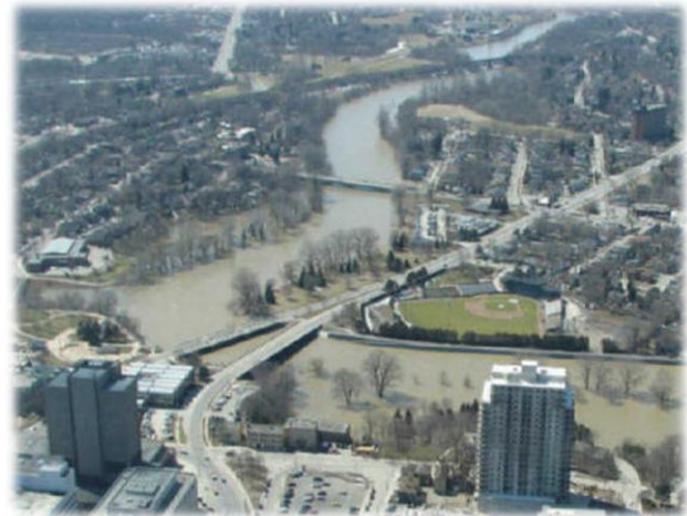
Figure 1.15: 2008 Flood (Main Branch)
