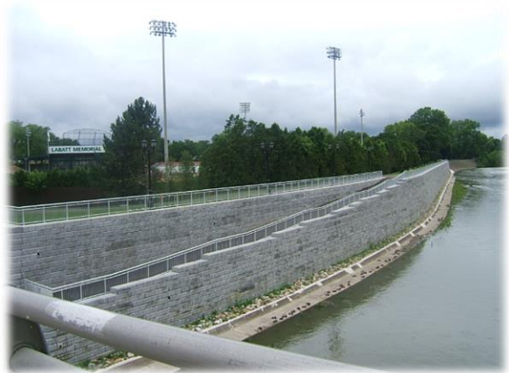
Figure 7.13: Phase 1 (from Queens Avenue Bridge)
