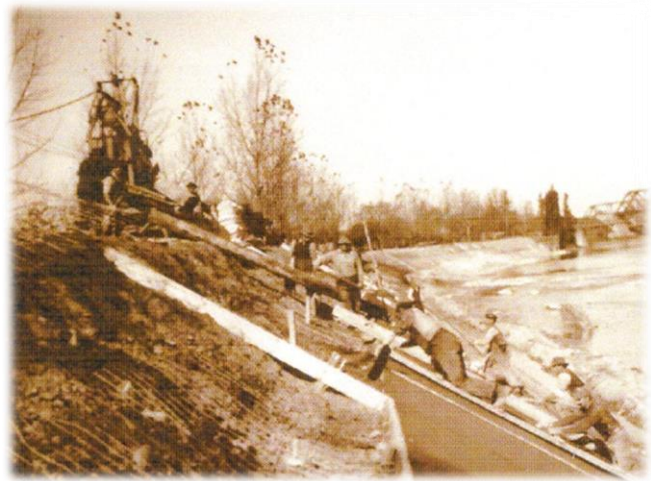
Figure 1.4: Construction of the Dyke
