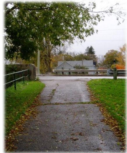
Figure 7.20: View West to the Wharncliffe Road North Crossing
