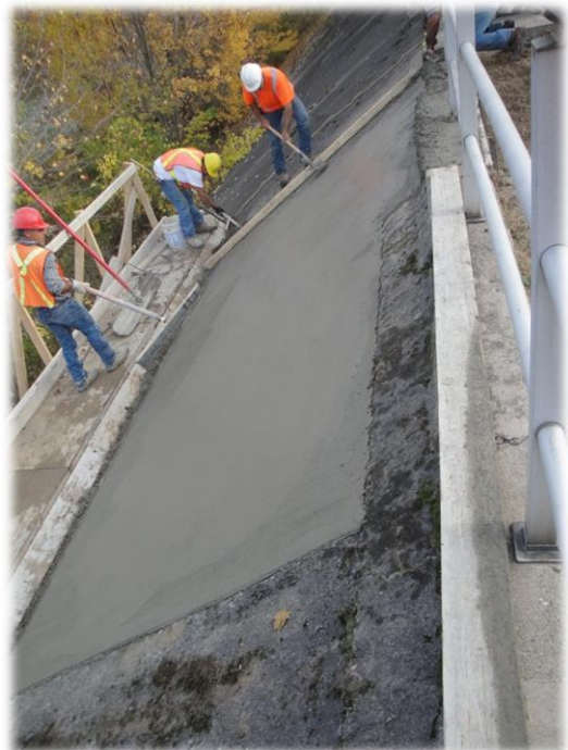
Figure 10.3: Panel Deficiency Repair
