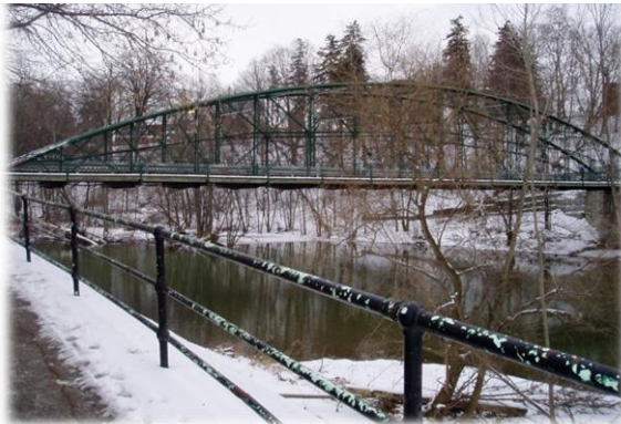
Figure 7.18: View of Blackfriars Bridge (from South)
