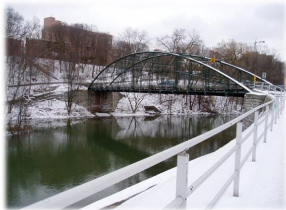
Figure 7.19: View of Blackfriars Bridge (from North)
