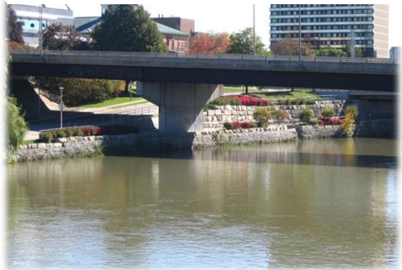
Figure 7.14: View of Queens Avenue Bridge
