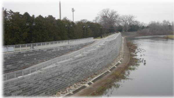
Figure 4.14: Phase 1 Structure (Pre-Cast Modular, Facing North)
