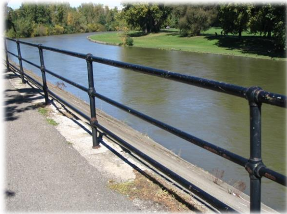
Figure 7.9: Existing Dyke Railing
