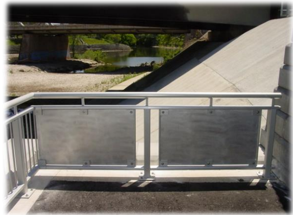
Figure 7.10: New Dyke Railing, Complete with Inserts
