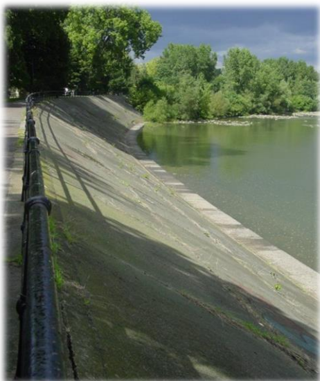
Figure 7.3: Natural Curve Observed in Existing Structure
