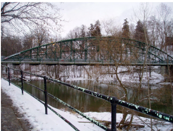
Fig. 4.24 View of Blackfriars Bridge from South.
