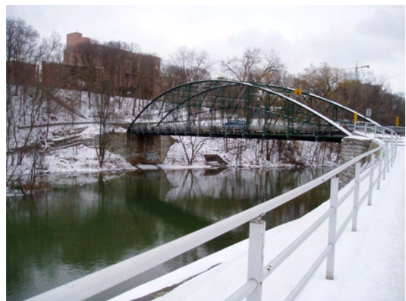
Fig. 4.25 View of Blackfriars Bridge from North.
