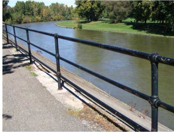
Fig. 4.14 Existing dyke railing.
