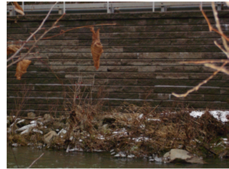
Fig. 4.4 Pre-cast wall material.
