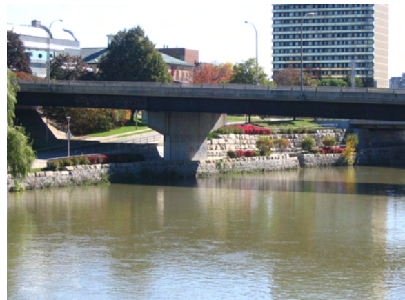
Fig. 4.20 View of Queens Avenue Bridge and the Fork of the Thames.
