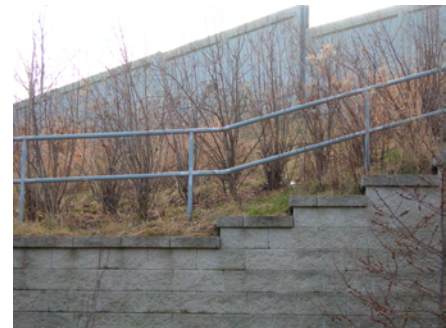
Fig. 4.5 Pre-cast wall material.
