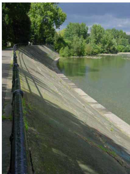
Fig. 4.6 Natural curve observed in existing structure.
