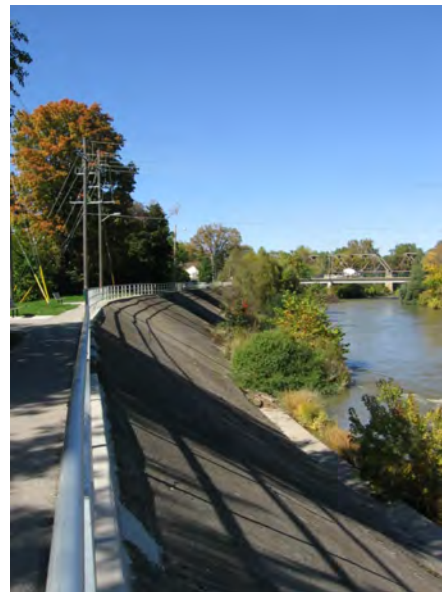
Fig. 2.1 View North towards Oxford Street Bridge.
