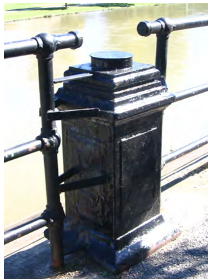
Fig. 4.12 Historic light base incorporated into existing dyke railing.
