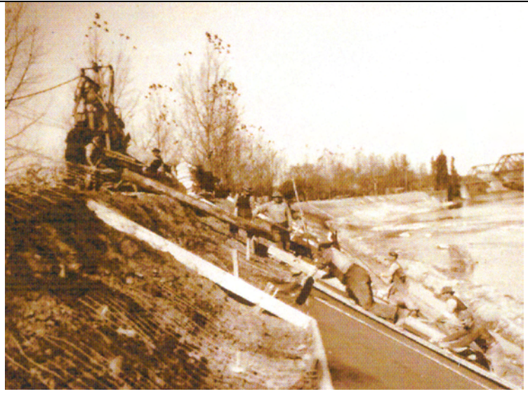
Fig -1 Photo from the 1930's showing the concrete Dyke being formed.
