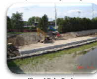
2007 Phase I Dyke Replacement
