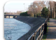
2005 Concrete Repair Program
