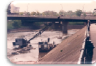
1980's Repair Work
