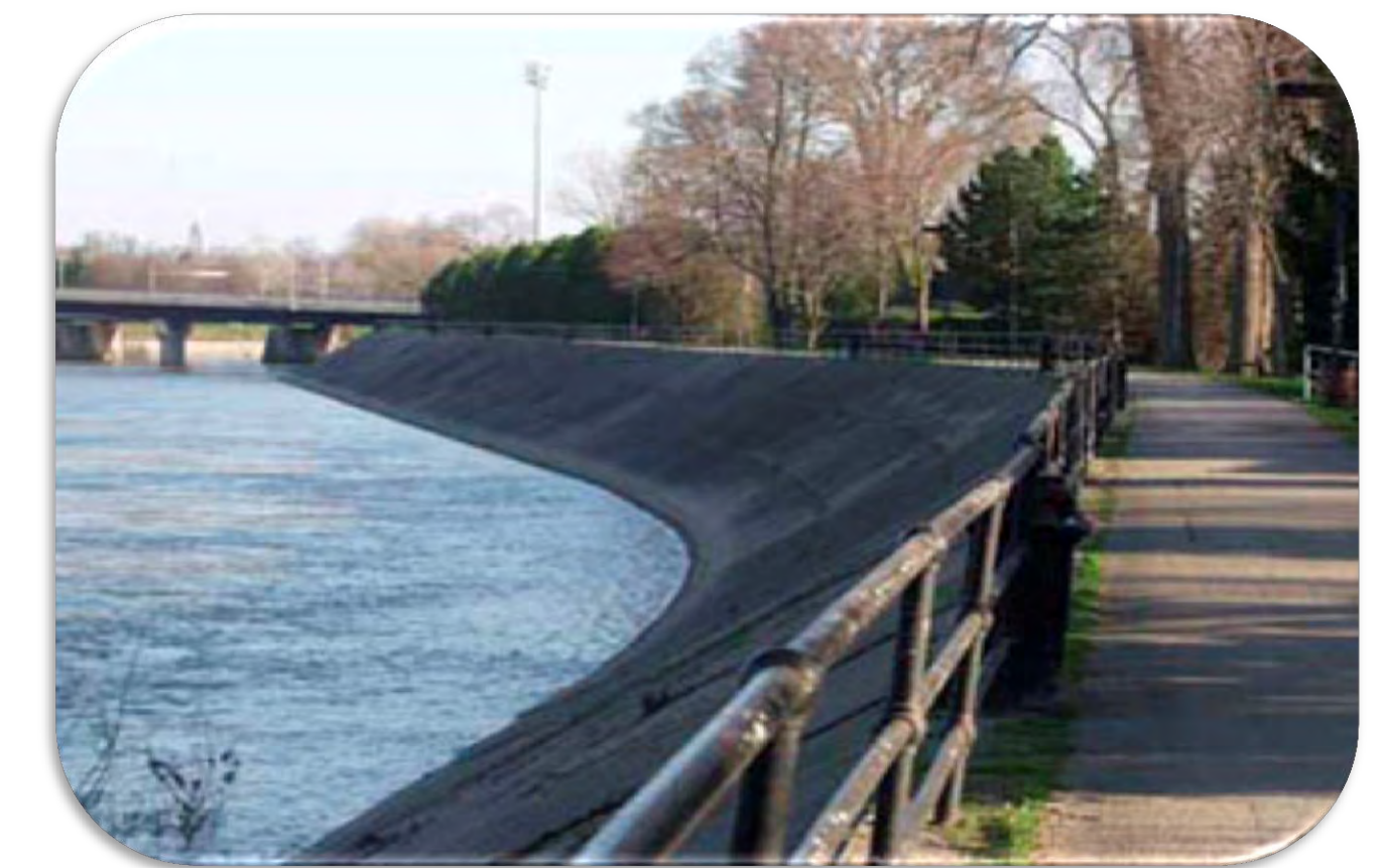
2005 Concrete Repair Program
