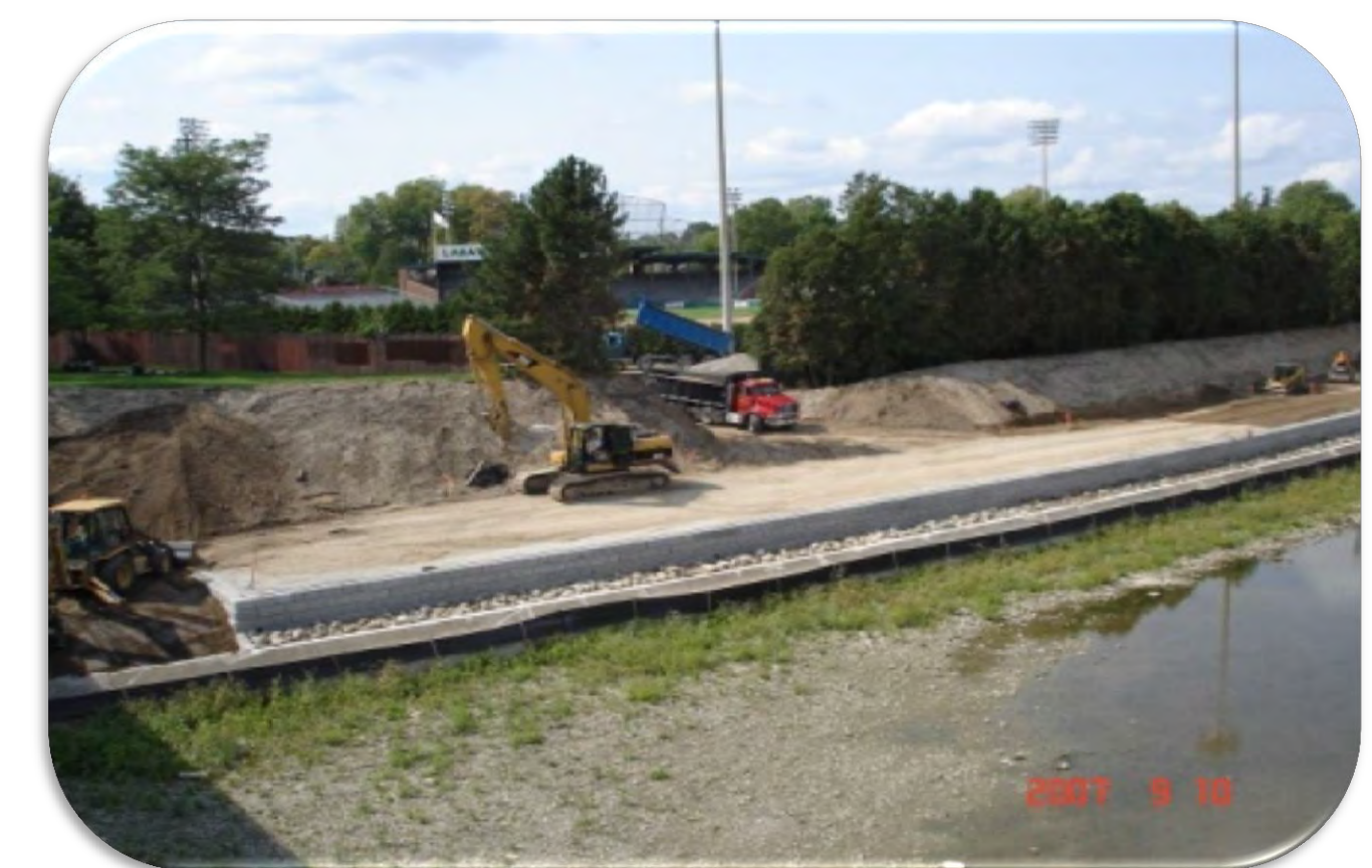
2007 Phase I Dyke Replacement
