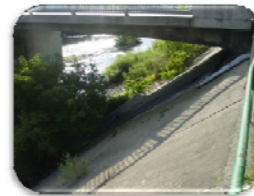
Vegetation at Toe of Dyke
