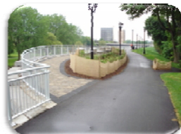
Top of Dyke Look-Out
