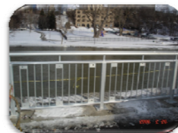
Provision of Tabs Along Railing
