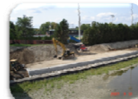
2007 Phase I Dyke Replacement
