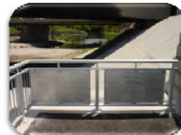
Panel with Tabs for Future Display Panels
