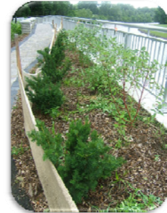
Top of Dyke Vegetation
