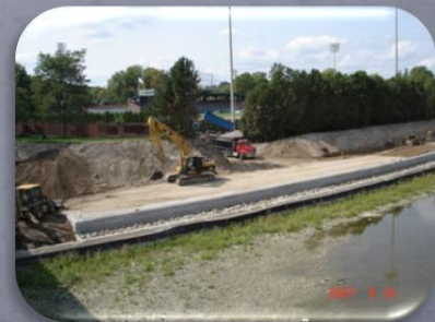
2007 Phase I Dyke Replacement
