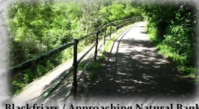
Blackfriars / Approaching Natural Bank
