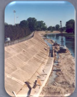
1980's Repair Work
