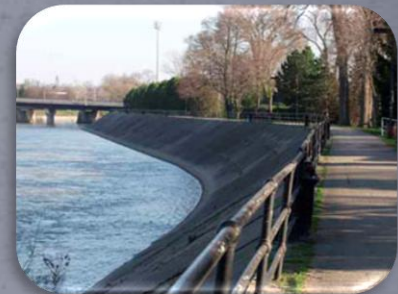
2005 Concrete Repair Program
