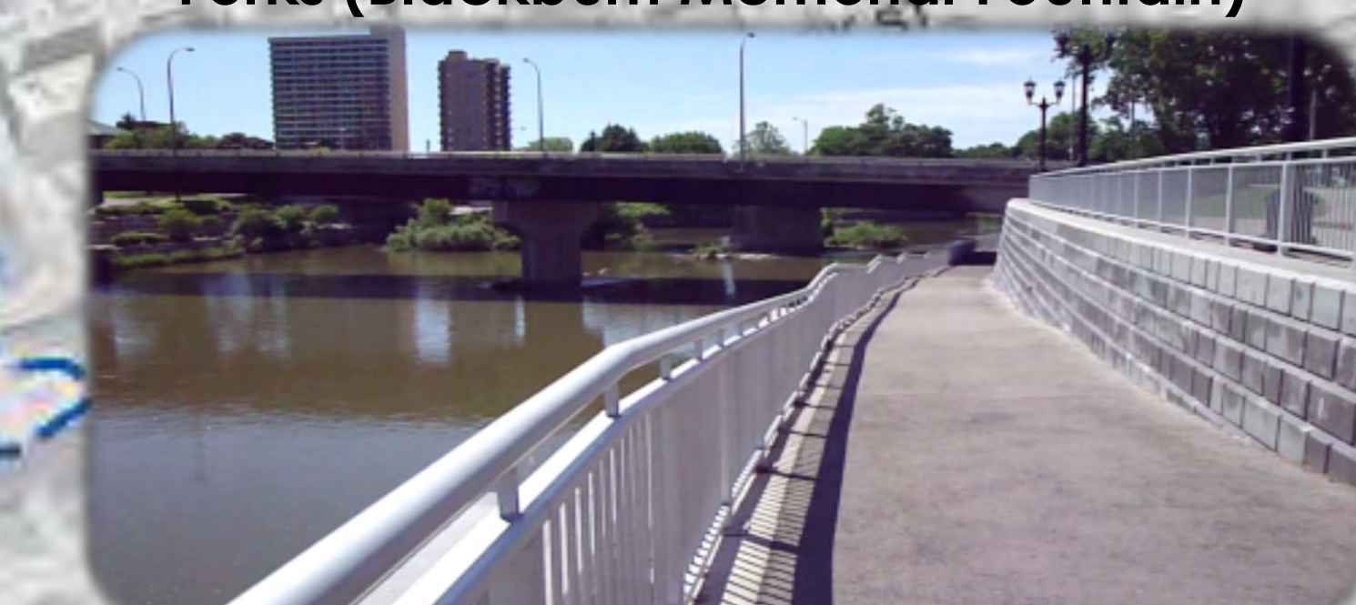
Labatt Park / Forks (Pedestrian Underpass)
