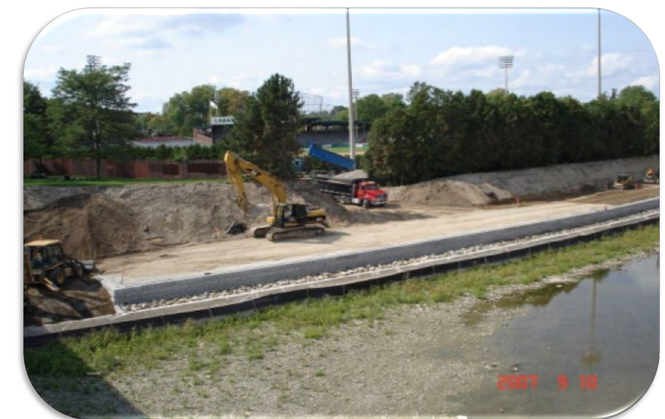
2007 Phase I Dyke Replacement
