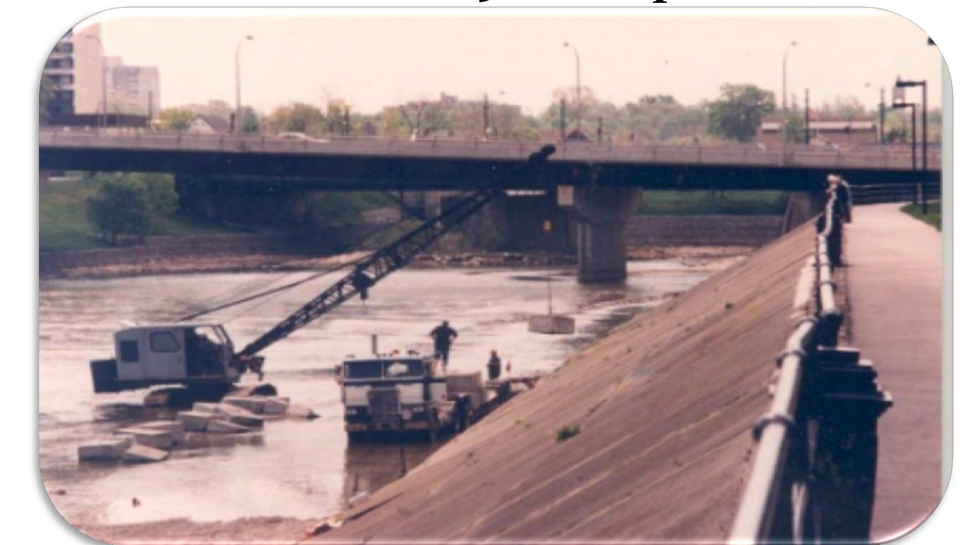
1980's Repair Work
