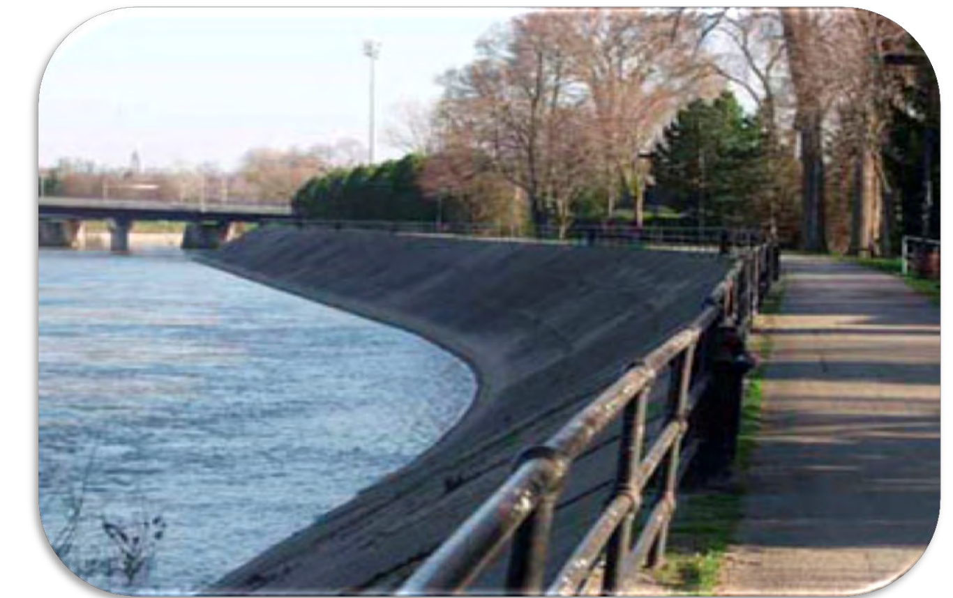
2005 Concrete Repair Program
