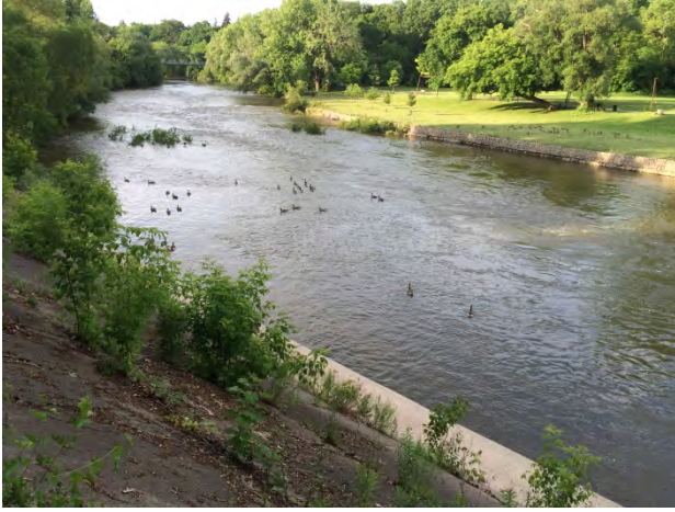
Photo 2-7 – Leslie Street Site (Vantage 1), June 13, 2015. River discharge 26.8 m 3 /s. Note calm conditions at toe of dyke (foreground).
