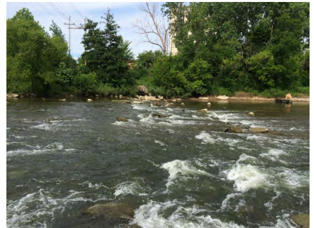
Photo 1-4 – On top of Ann Street Weir looking eastward from right bank to left bank. Flow to right.
