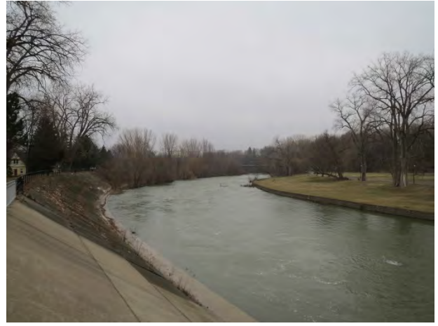
Photo 2-2 – Leslie Street Site (Vantage 1), April 8, 2015. River discharge 38.0 m 3 /s. Some turbulence evident along dyke toe.
