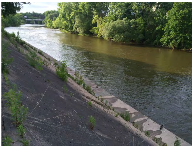
Photo 1-5 – Ann Street Weir, June 13, 2015. River discharge 26.8 m 3 /s. Vantage is approximately 100 m downstream of vantage of photos 1-1 to 1-4.
