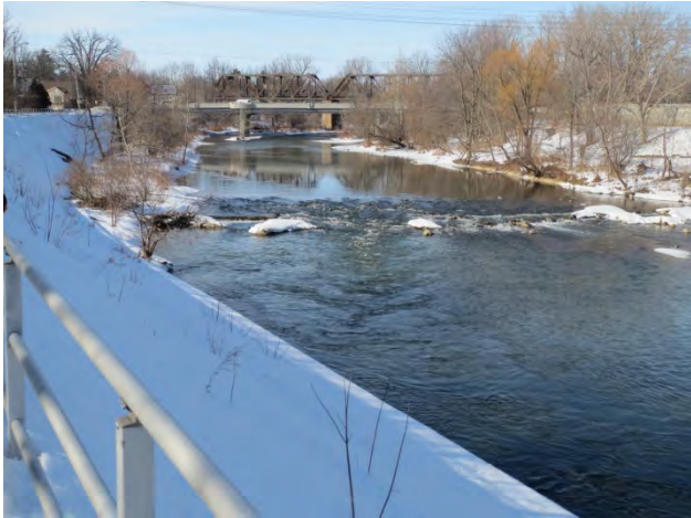
Photo 1-1 – Ann Street Weir showing flows coming off weir toward the dyke (foreground). March 12, 2015. River discharge: 3.9 m 3 /s.
