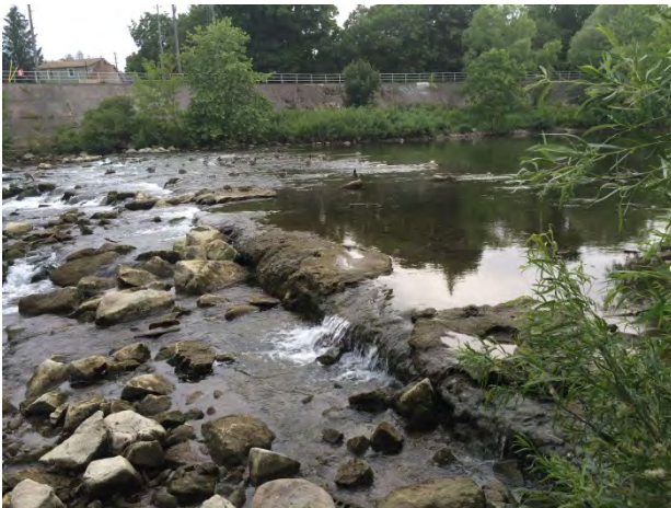
Photo 1-5 – On top of Ann Street Weir looking concrete structure and riprap. View toward right bank, flow to left.
