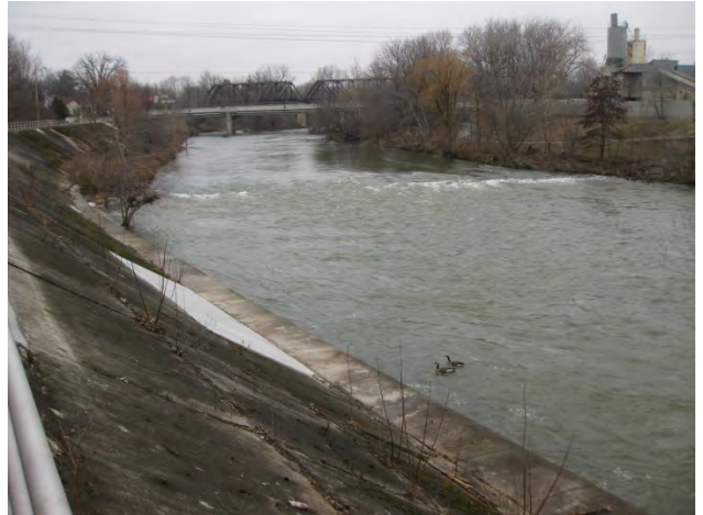
Photo 1-2 – Ann Street Weir, April 8, 2015. River discharge 38.0 m 3 /s.
