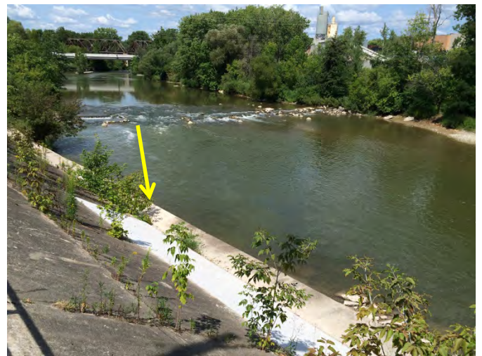
Photo 1-6 – Ann Street Weir, August 22, 2015. River discharge 5.4 m 3 /s. Flow vector intercepts bank approximately 40 m downstream of weir (arrow).
