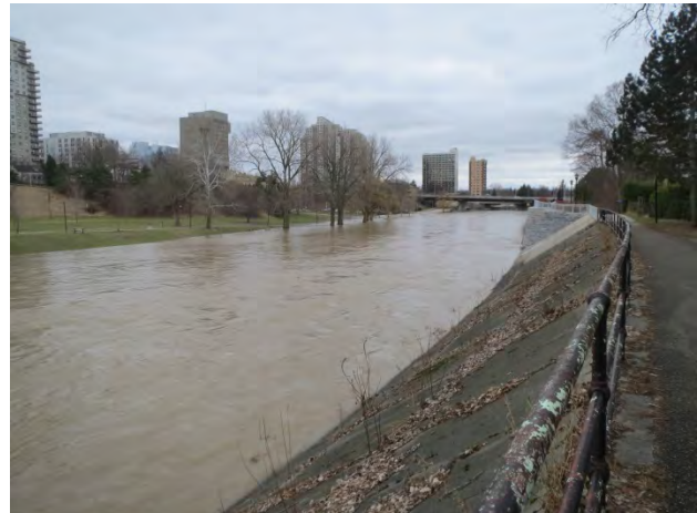
Photo 2-4 – Leslie Street Site (Vantage 2 - downstream), April 10, 2015. View of downstream section of compound pool. Boils on water surface near the dyke toe indicate turbulence (kolks) and high shear.
