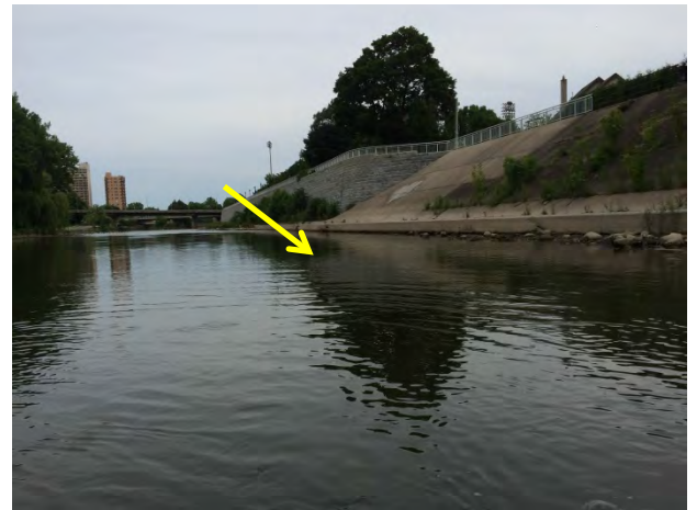
Photo 2-4 – Leslie Street Site looking downstream. The deepest part of the scour pool is located at the transition from sloped to vertical dyke wall at the foot of Rogers Avenue (arrow).
