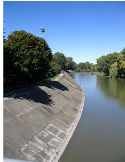
Fig. 4.19 West side of dyke, looking North from the Queen St. Bridge.
