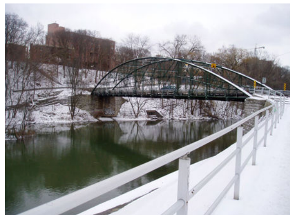
Fig. 4.25 View of Blackfriars Bridge from North.
