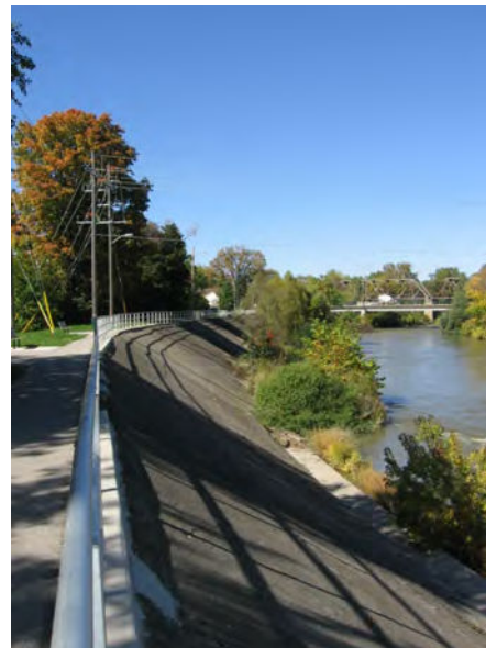
Fig. 2.1 View North towards Oxford Street Bridge.
