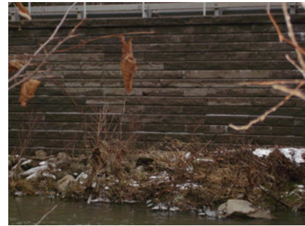
Fig. 4.4 Pre-cast wall material.
