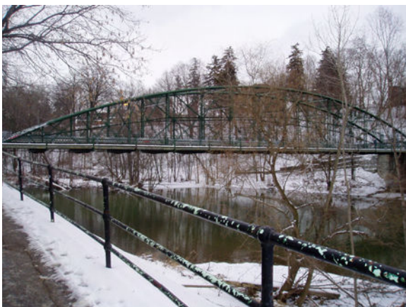
Fig. 4.24 View of Blackfriars Bridge from South.
