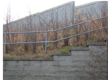
Fig. 4.5 Pre-cast wall material.
