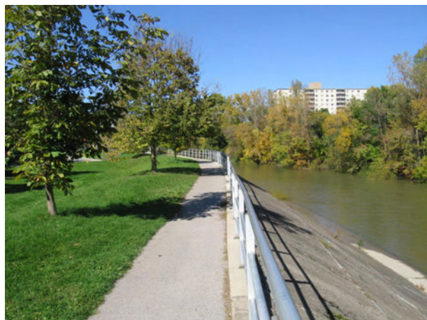
Fig. 2.2 View North-East from Blackfriars Bridge.
