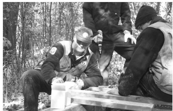
Boardwalk construction near Spettigues Pond
