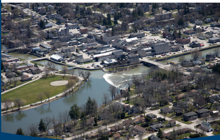
A 550 metre long floodwall, constructed in 1990 where Trout Creek (middle left) enters the North Thames River (lower left to middle right), protects historic downtown St. Marys from flooding up to the floodwall's designed level of protection (100 year flood).
