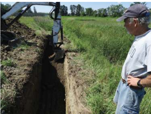
Step 1: Trench is dug within riparian buffer strip.
