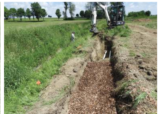
Step 3: Trench is backfilled with woodchips
